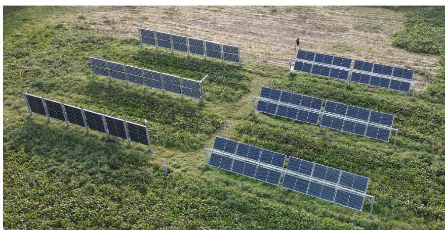
Figure 1: Overview of two agrivoltaic systems in Grembergen: a fixed vertical system (left) and a horizontal single axis tracking system (right).
