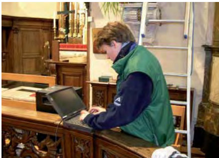
An inspector is making notes about the condition of the building using a laptop.
