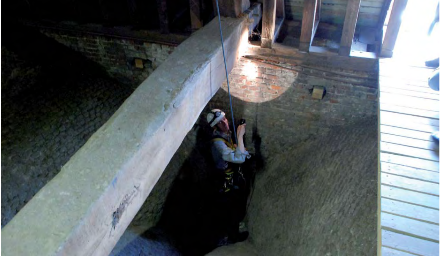
Inspecting a church roof
