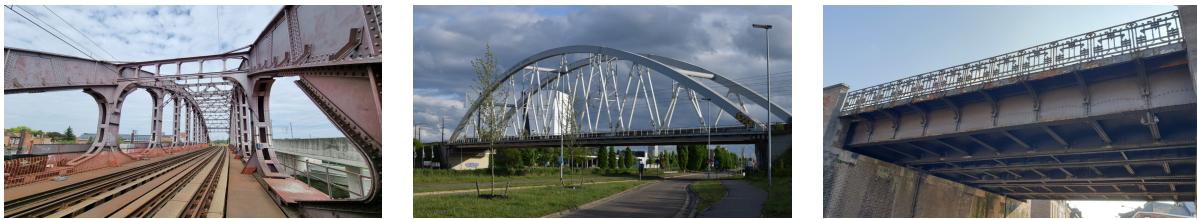
Figure 1: Left: The Vierendeel arch bridge (Mechelen, Belgium). Center: The KW51 tied-arch bridge (Leuven, Belgium). Right: The Nieuwebrugstraat riveted beam bridge (Ronse, Belgium).
