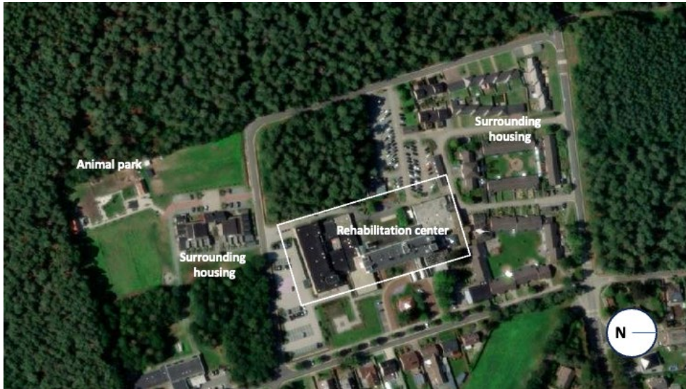
Figure 1. Aerial view of the rehabilitation center and its surroundings (source: open streetmap, with additions by the first author)
