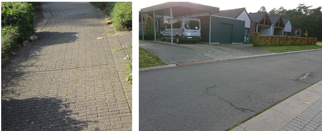
Figure 5. Detailing of outdoor environment (Left: Small unevenness in pavement. Right: efforts made for optimal accessibility e.g. no or covered gutter)
