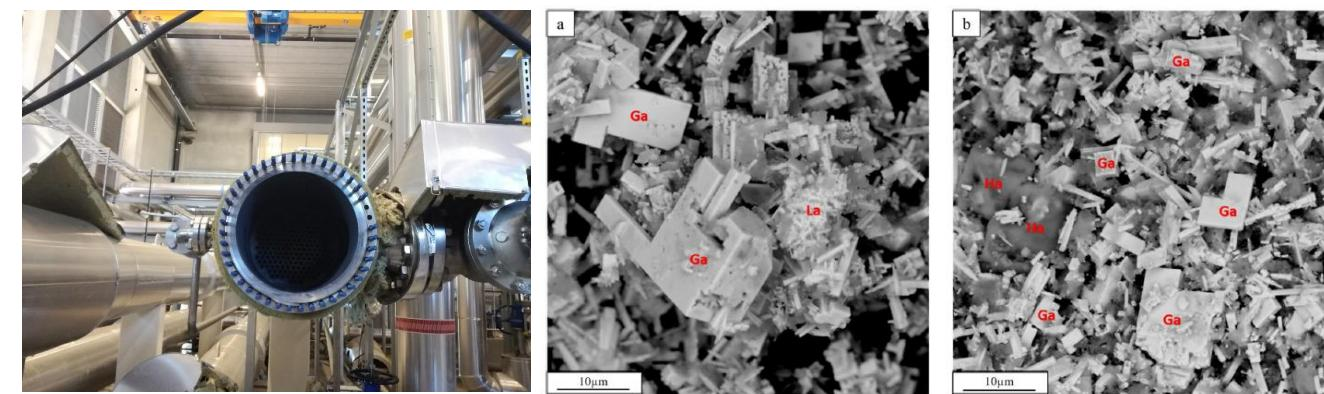
Fig 1. Heat exchanger (HEX) of the Balmatt geothermal installation; SE images (SEM) of mineral scales in the HEX of the Balmatt geothermal installation (taken from Pauwels et al., 2021)
