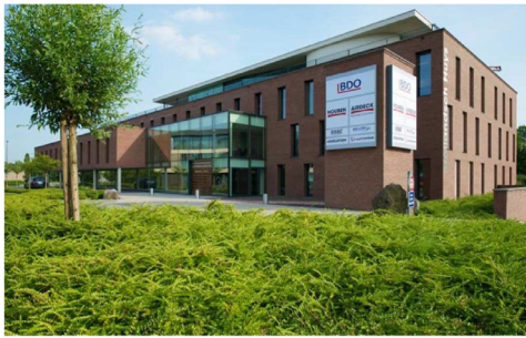
(a) Building from outside.
