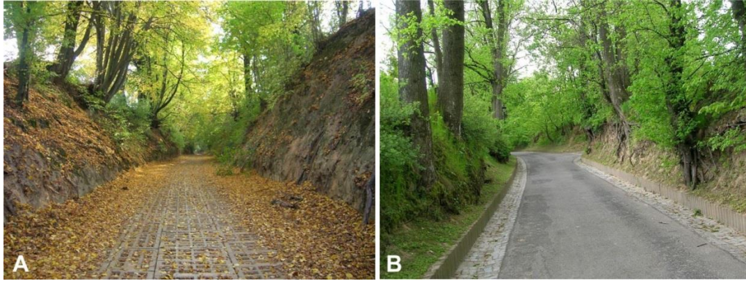
Figure 11. Different methods of paving bottoms of sunken lanes. A - openwork concrete slabs (Nałęczów Plateau, E Poland, loess), B – asphalt (Roztocze Region, E Poland, loess). (Photo: J. Rodzik).
