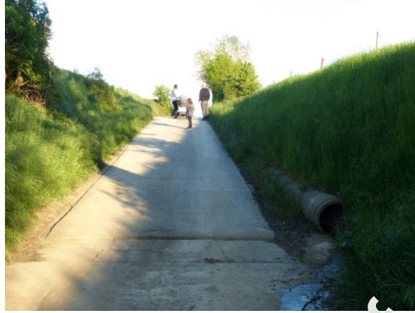
Figure 12. Sunken lane converted into a temporary flood retention pond by installing a concrete dam and a pipe to allow for bypass flow (Sluizen, Belgium 2019) (Photo: J. Poesen).
