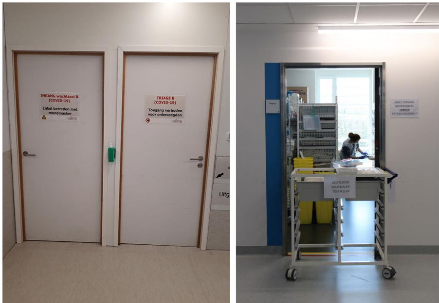
Figure 3. A waiting room in Hospital A was split adding 2 additional spaces: a separate waiting room for (potential) Covid patients and a triage space (left). A nurses' station indicating only those who have not had direct (Covid) patient contact may enter (Hospital F, right).
