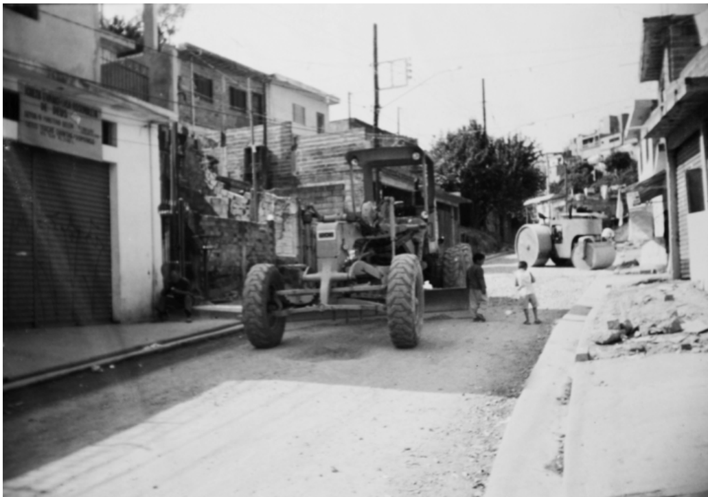
Figure 8. Paving of a Street in Guapira I, 1999. (Photo by Neto)
