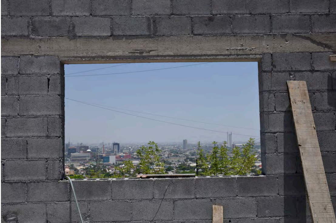
Figure 8. A window frames the large inside city. (Source: author)
