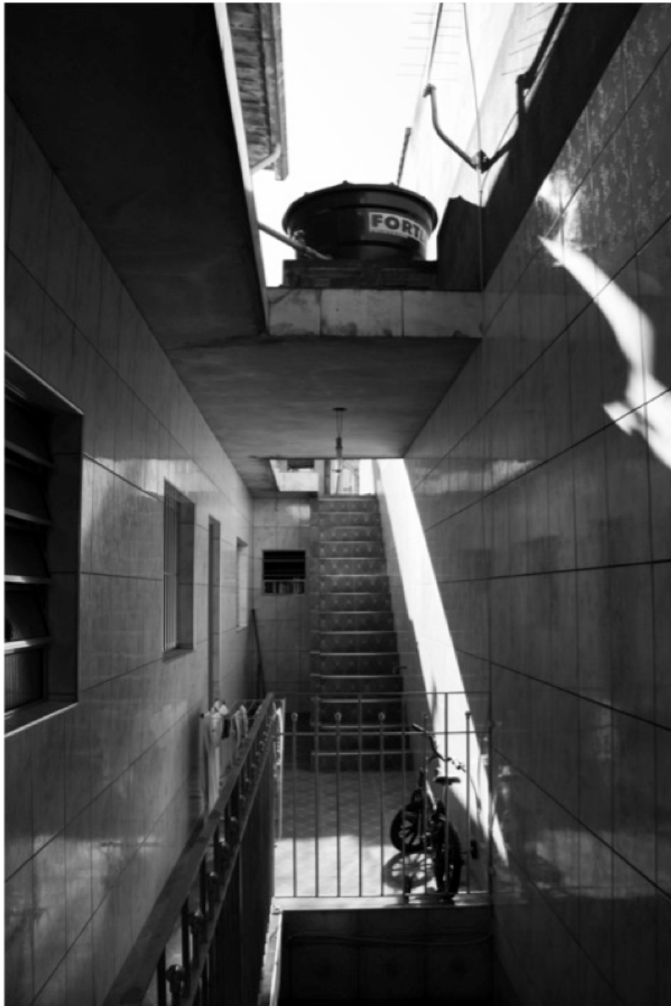
Figure 6. The External Staircase of Neto's House. (Photo by the Author)
