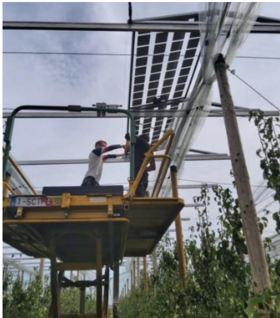
Figure 10: Photograph taken during the installation phase of the agrovoltaic system at Bierbeek.
