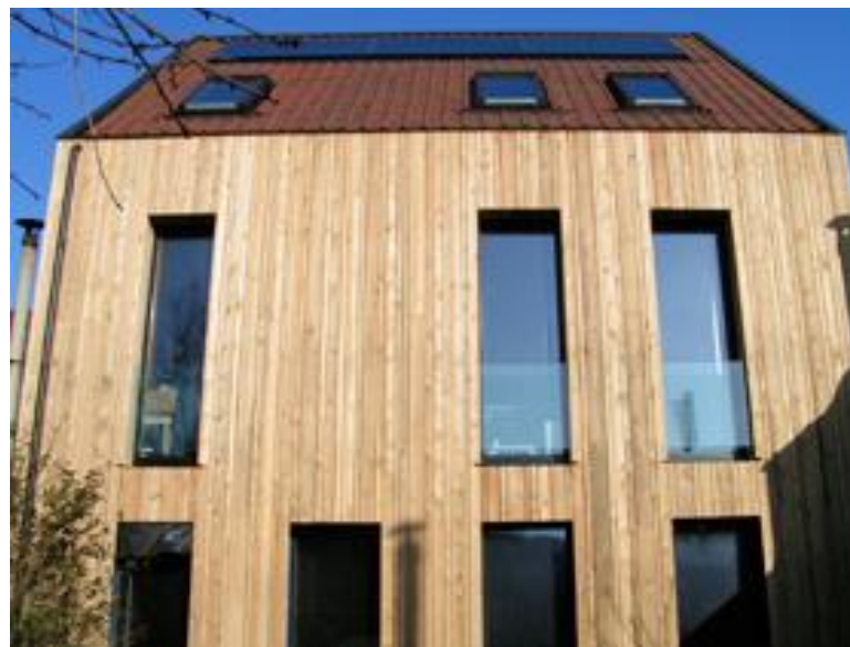
gevelbekleding in hout
