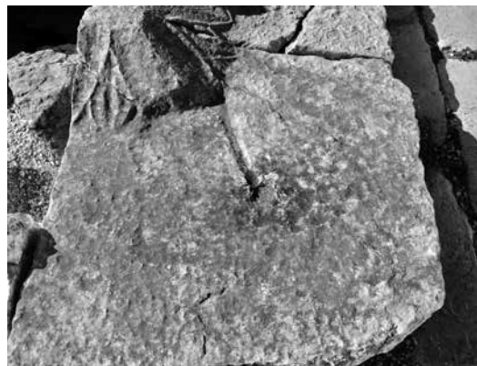
Fig. 5 Northwest corner of the canopy roof
