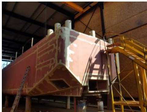
Figure A1. Construction phase 360-degree-steerable four-channel stern thruster on a CEMT-I.
