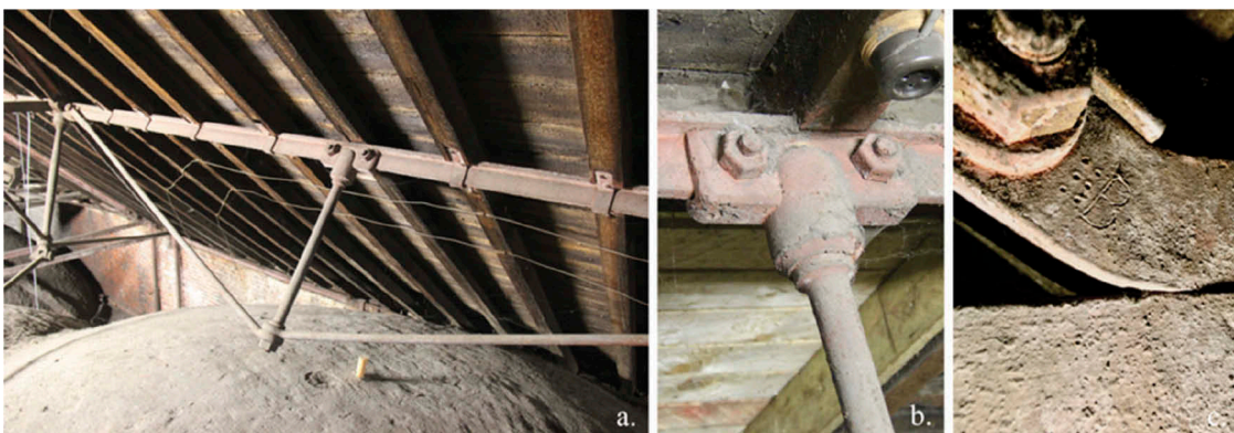
Figure 5. St. George's construction details. (a) trussed-beam bracing, (b) screwed assembly, (c) assembly mark: "B" and 6 dots (pictures R. Wibaut and I. Wouters).
