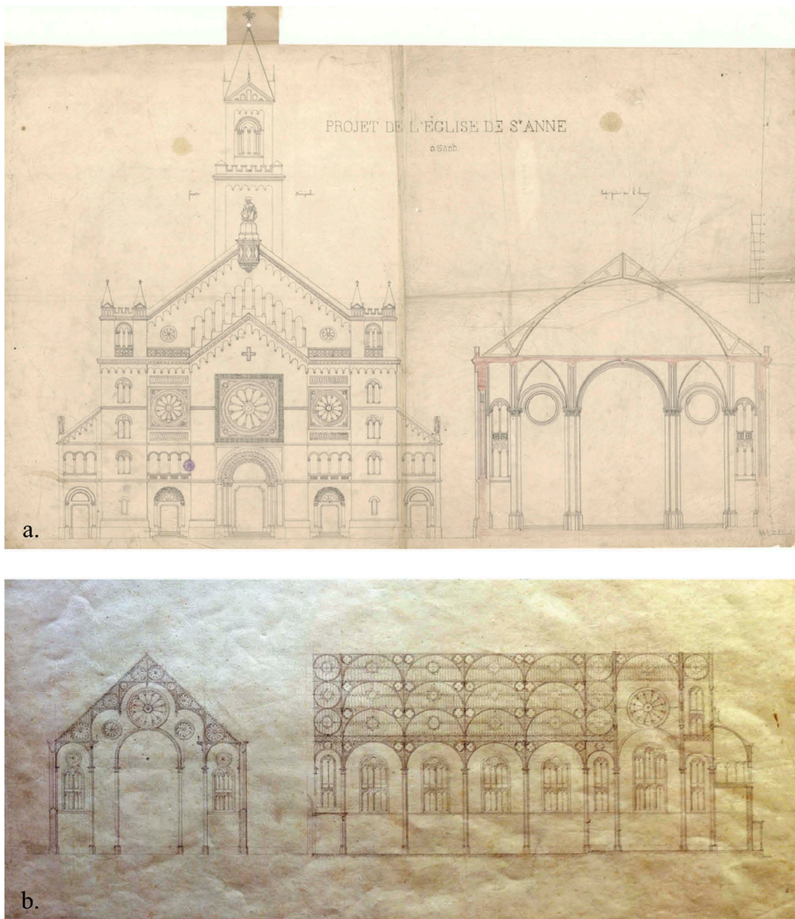
Figure 7. L. Roelandt's preliminary design for the St. Anne's Church. (a) Hidden cast-iron trusses (City Archives of Ghent, Atlas Goetghebuer, L135/11). (b) Visible cast-iron structure (Archives of the Library of the University of Ghent, BIB.ARCH.003566).
