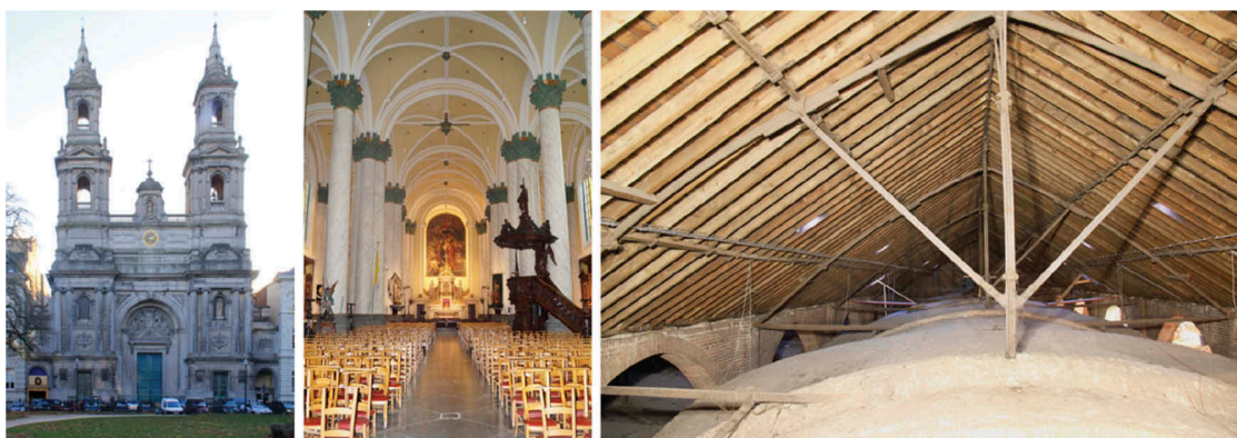
Figure 2. St. Joseph’s Church (1842–49) in Brussels. Exterior, interior and trusses (c. 1845) (pictures R. Wibaut and I. Wouters).
