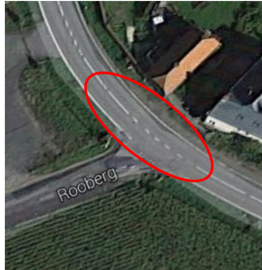
Figuur 40: Dangerous situation
