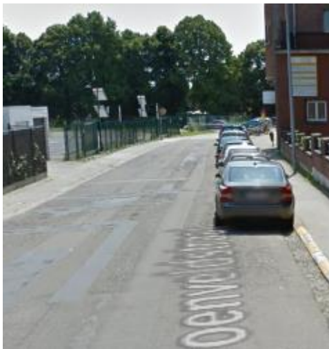
Figuur 41: Dangerous situation
