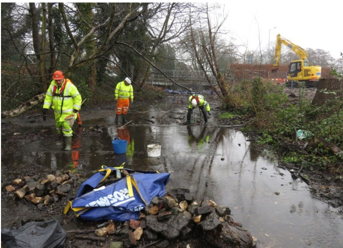
Figure 8e. partially dewatered channel with searchable piles of stones placed for crayfish leaving the dewatered bridge zone (plus one of the bags of collected beer bottles)
