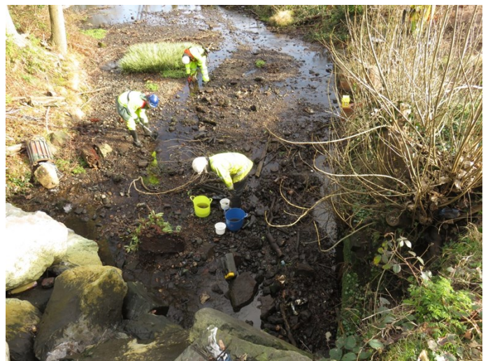
Figure 8c. view of de-watered channel downstream from the bridge
