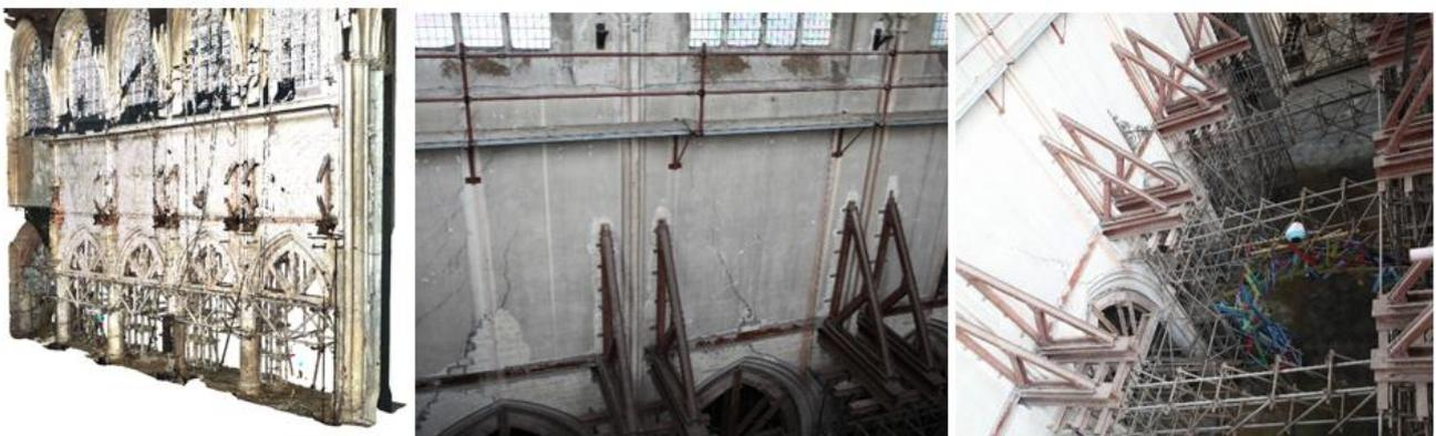
**Figure 4.** Overview northern naïve wall point cloud (left), settlement-induced cracks in the imagery (mid) and the occlusions caused by the shoring system in the church (right).
