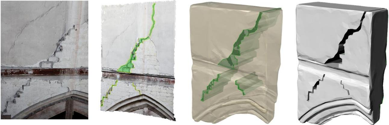
**Figure 3.** Overview Crack detection and modelling: Crack imagery (a), Textured Mesh with manually modelled crack geometry in green (b), Collision in green between Crack geometry and Volumetric Mesh (c) and the Crack representation in the final model (d).
