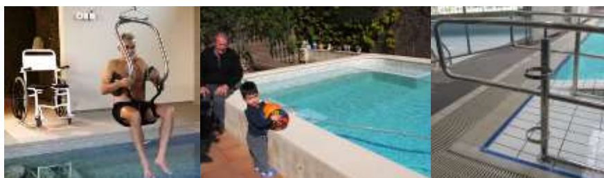
Figs. Left: 1. Ceiling-mounted pool lift; Centre: 2. Private pool in Spain with transfer bed; Right: 3. Public pool in Australia with cane holder (credits: 1. H.-M.; 2. M. B.-E.; 3. F. D.).
