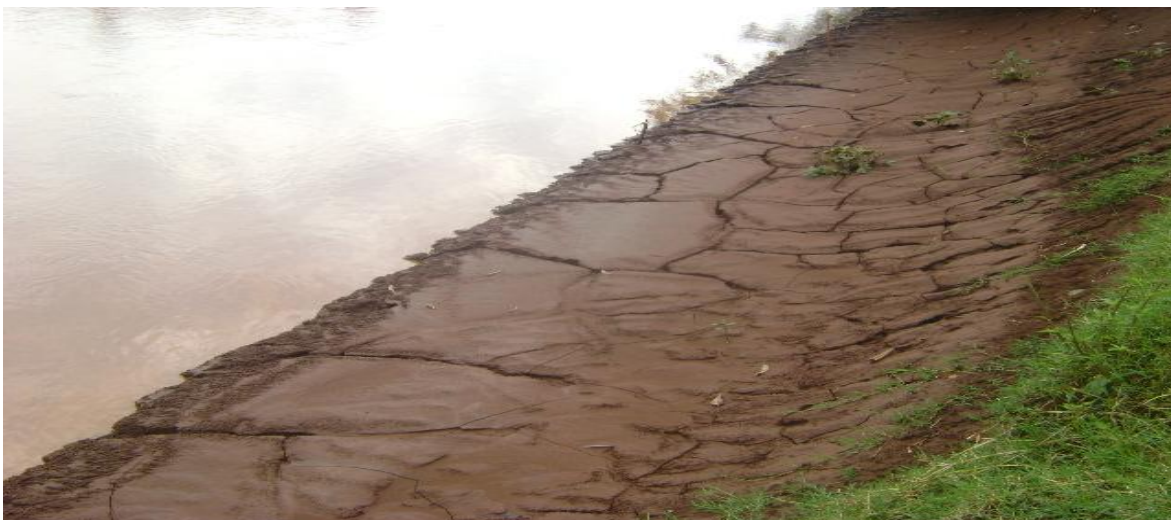
Figure 1. Sediment deposited by from Gilgel Abay River at Chimba wetland (July 2014)
