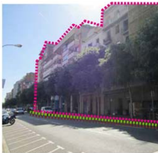
New exposed facade
