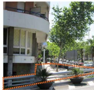
Detail on the level difference in the South West corner
