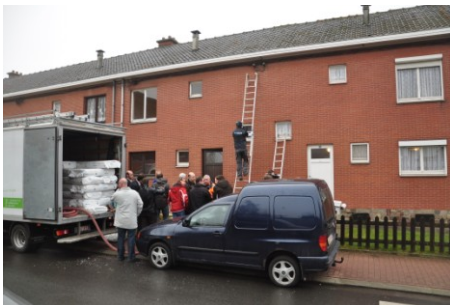
FIG 3. Investigated terraced house in Herstal, Belgium. (a) Front façade; (b) Garden façade.
