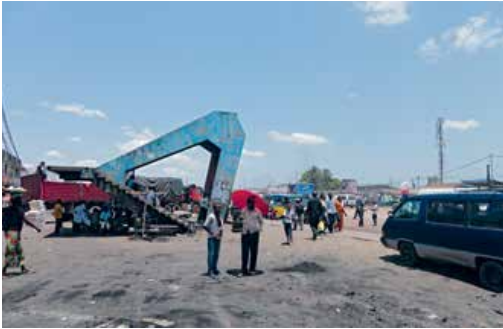
Remainder of pedestrian bridge along the Boulevard Lumumba.
