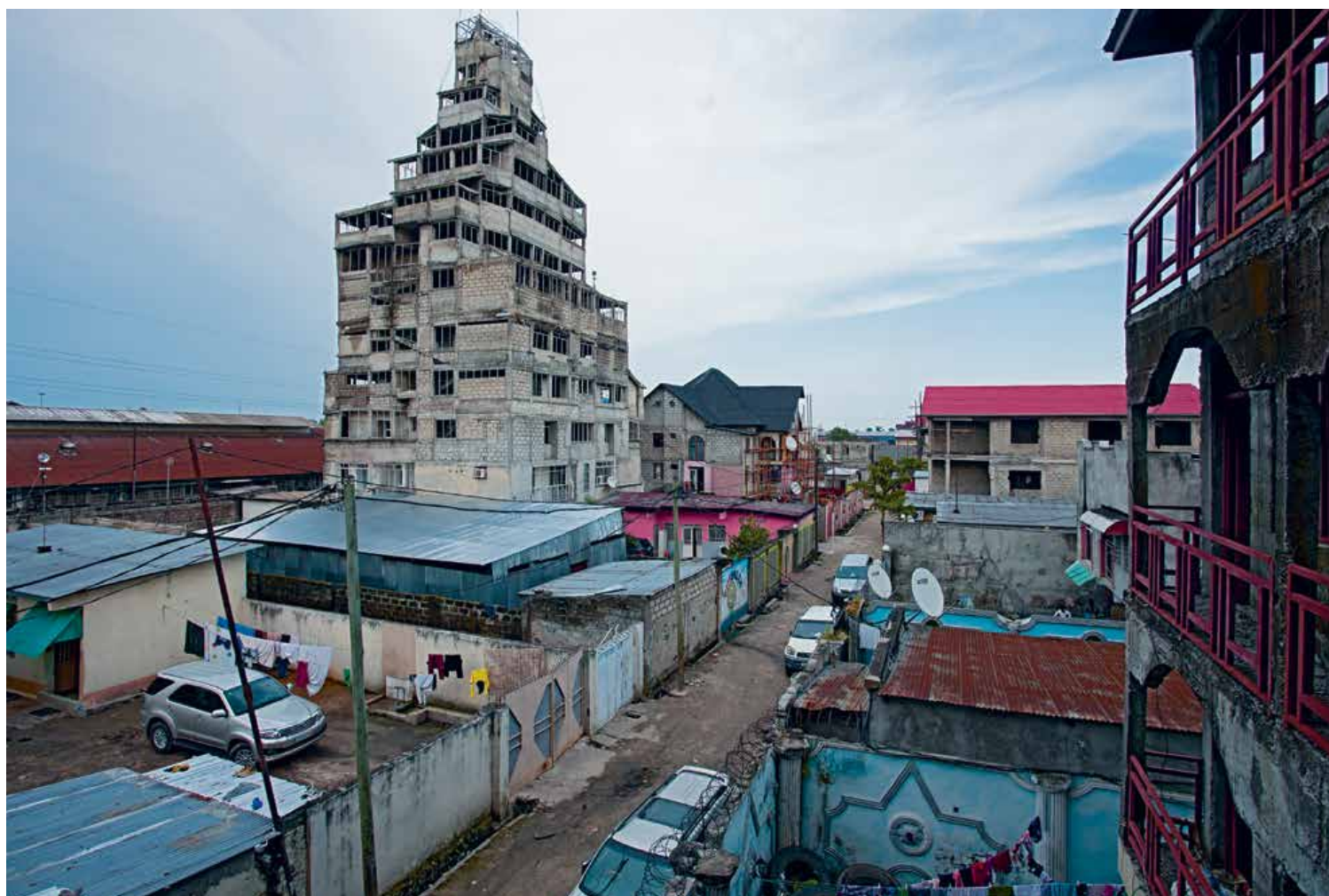
'The Tower', local skyscraper under construction. Photo: Municipality of Limete, March 2015
