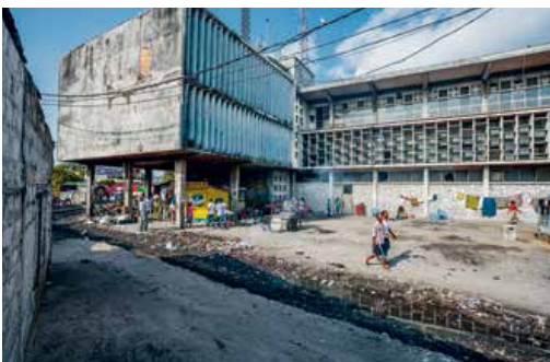
Constructed in the mid-1950s, the site Cielux OCPT (Office Congolais de Poste et Télécommunication), colloquially known as 'the Building' (le Bâtiment), is located in Sans Fil ('Wireless'), a neighbourhood of the populous municipality of Masina. The Cielux site is a branch of Kinshasa's central post office. A grand modernist L-shaped building, it used to house a section of the national radio, and it functioned as an outgoing relay station for international telephone and telegraph communications (hence the name 'wireless' which is now used to refer to the neighbourhood as a whole). Today the building is squatted by some 300 people, mostly unpaid government employees of the Ministry of Telecommunications. Photo: Site Cielux, Municipality of Masina, March 2013
