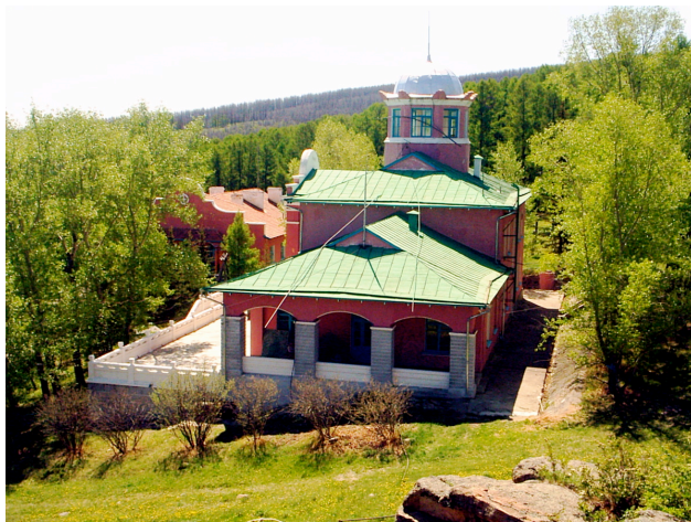
Fig.1 – Main building at Khureltogot Observatory
