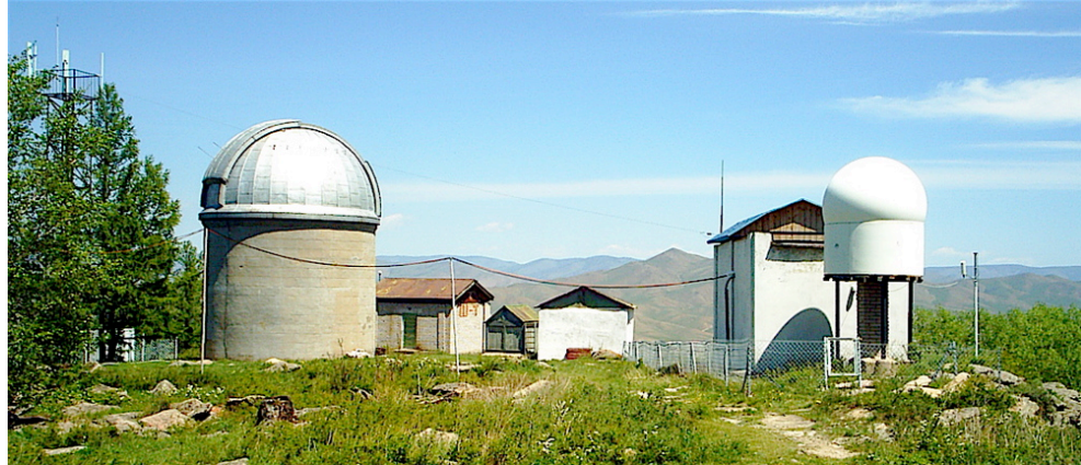
Fig.2 – A few of the buildings at Khureltogot observatory
