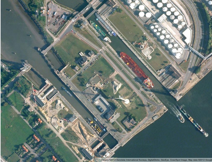
Figure 2.3: Photograph of the Boudewijn - Van Cauwelaert lock complex in the Port of Antwerp, Belgium. (©2012 Google, Aerodata International Surveys, DigitalGlobe, GeoEye, Cnes/Spot Image, Map data ©2012 Google)
