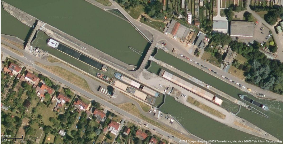
Figure 2.1: Photograph of the Wijnegem lock on the Albertkanaal in Belgium. (©2009 Google, TerraMetrics)
