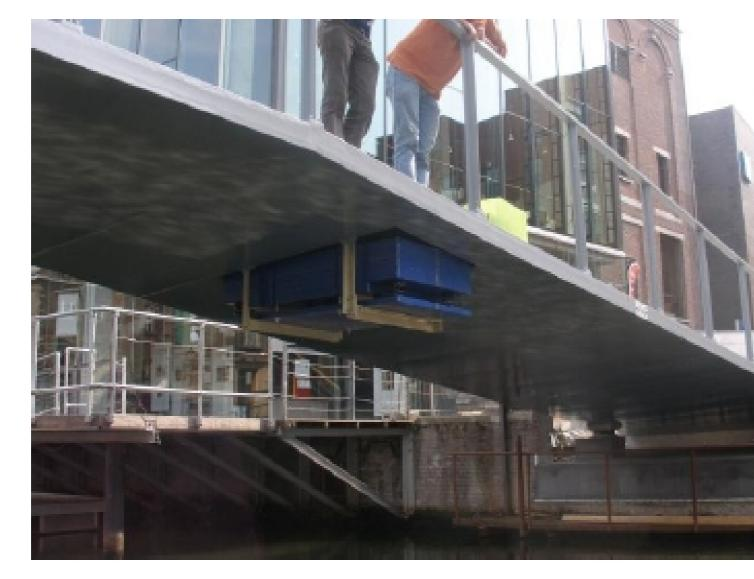
Goal: Minimize the vibration by tuning the stiffnesses and the damping coefficients of the four dampers. (8 design parameters)
