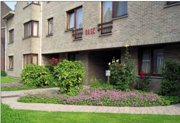
Figure 7 The articulated facade of Luc's apartment gives a welcoming impression.
