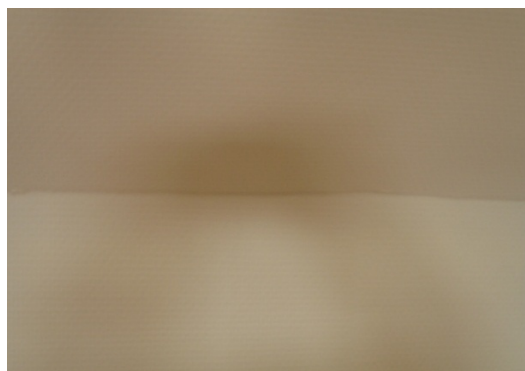
Figure 11. Picture of the boundary between the sloping ceiling and the wall
