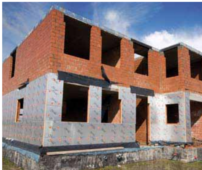
foto Recticel Insulation
