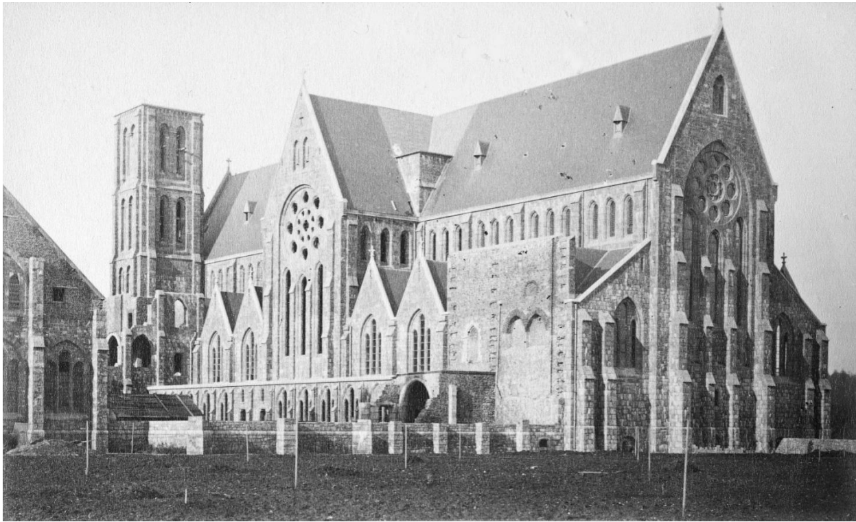
Fig. 8. Maredsous, abbey church under construction, ca 1880 (Archives of the Abbey of Maredsous).
