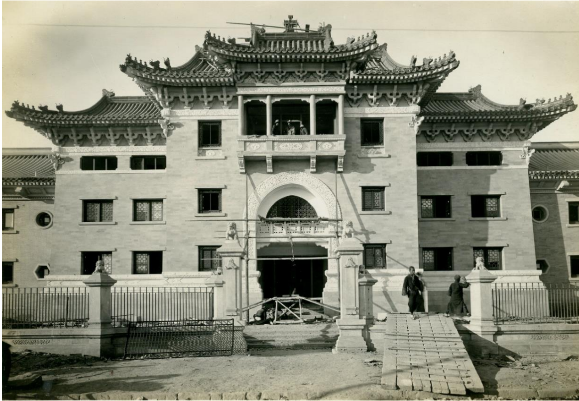
Fig. 1. Beijing, Fu Jen Catholic University of Peking, main entrance, A. Gresnigt, 1930 (Archives of the Abbey of Maredsous).
