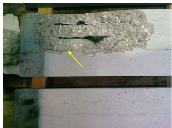
Fig. 3 Surfaces of concrete specimens exposed to fire. Upper sample: serious damage/spalling indicated with the arrow, reference concrete with only PP fibers ( 2 \text{ kg/m}^3 ). Lower sample: without any spalling, concrete containing SAP ( 1.93 \text{ kg/m}^3 ) and PP fibers ( 2 \text{ kg/m}^3 )
