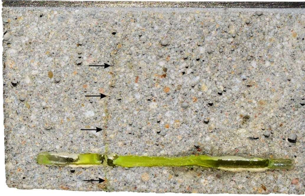
Fig. 15. Mortar specimen with mortar removed from the side up to the location of a capsule (length approximately 55 mm) showing that most of the PU was retained in the capsule. Arrows indicate the location of the crack.
