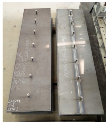
Figure 1: Shear studs in place before welding (Anon., sd) (a), scheme of the studied system (b) and specimens for four-point bending test before concreting (left: unwelded, right: welded)
