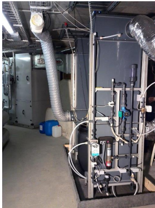
Figure 14: Prototypical device for air drying recirculation in the greenhouse of the Botanical Garden Berlin.
