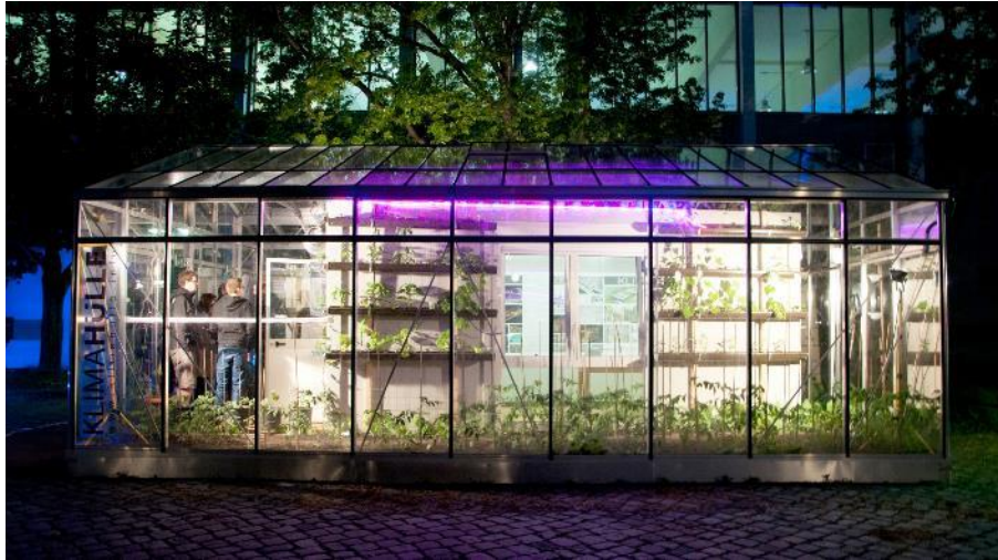
Figure 12: Greenhouse attached to a building for testing the Watergy absorber.
