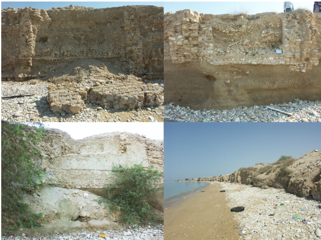
Figure 9. Remains along the beach between Site D and Site B, of dry-laid constructions, plastered surfaces including moulded decoration, traces of wooden ceiling beams, narrow partitions and stone flooring indicating interior spaces of buildings that once extended further towards the beach. (Photos: A. Trakadas)
