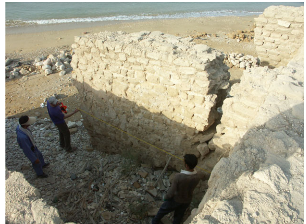
Figure 5. A seaward-facing buttness (marked with an 'X' in Fig. 4) on the southern side of the Congregational Mosque (Site B) clearly showing the impact of erosion. (Photo: A. Trakadas)
