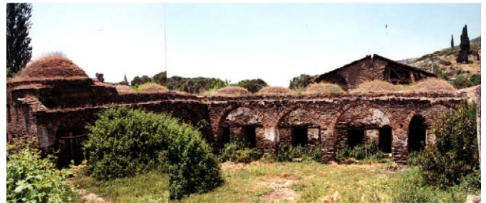
Fig. 4. Local construction technique composed of rubble stone, brick and mortar in random bond of Birgi Derviş Ağa Madrasa.
