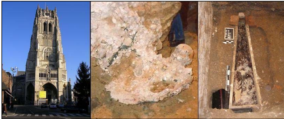
Fig.3 -- Left: tower of Our Lady's Basilica at Tongeren (Belgium) Middle: unwanted "consolidation" of a skeleton caused by the pronounced fluidity in time of the injected cement based grout (phase I) Right: sarcophagus next to the chain wall (excavated in phase II)
